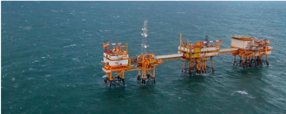
Figure 2-29: North Sea gas production platform L10-A of ENGIE (ENGIE, 2016)
