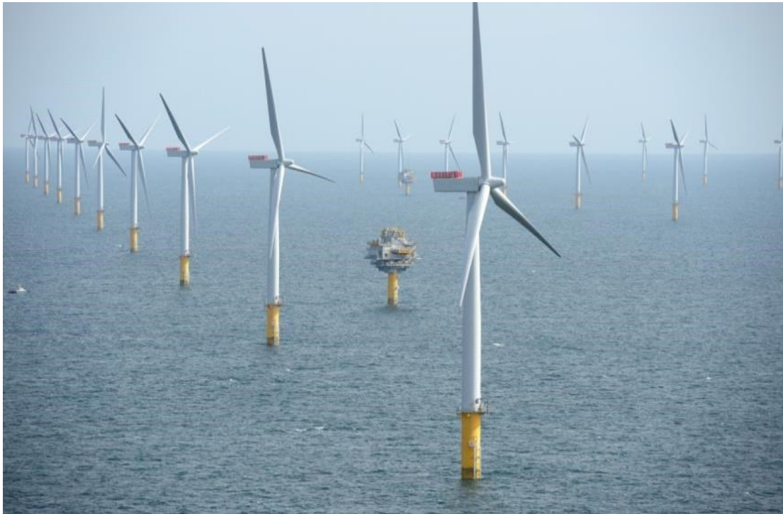
Figure 2-27: (left) Offshore wind park (Pettersen & Statoil)
