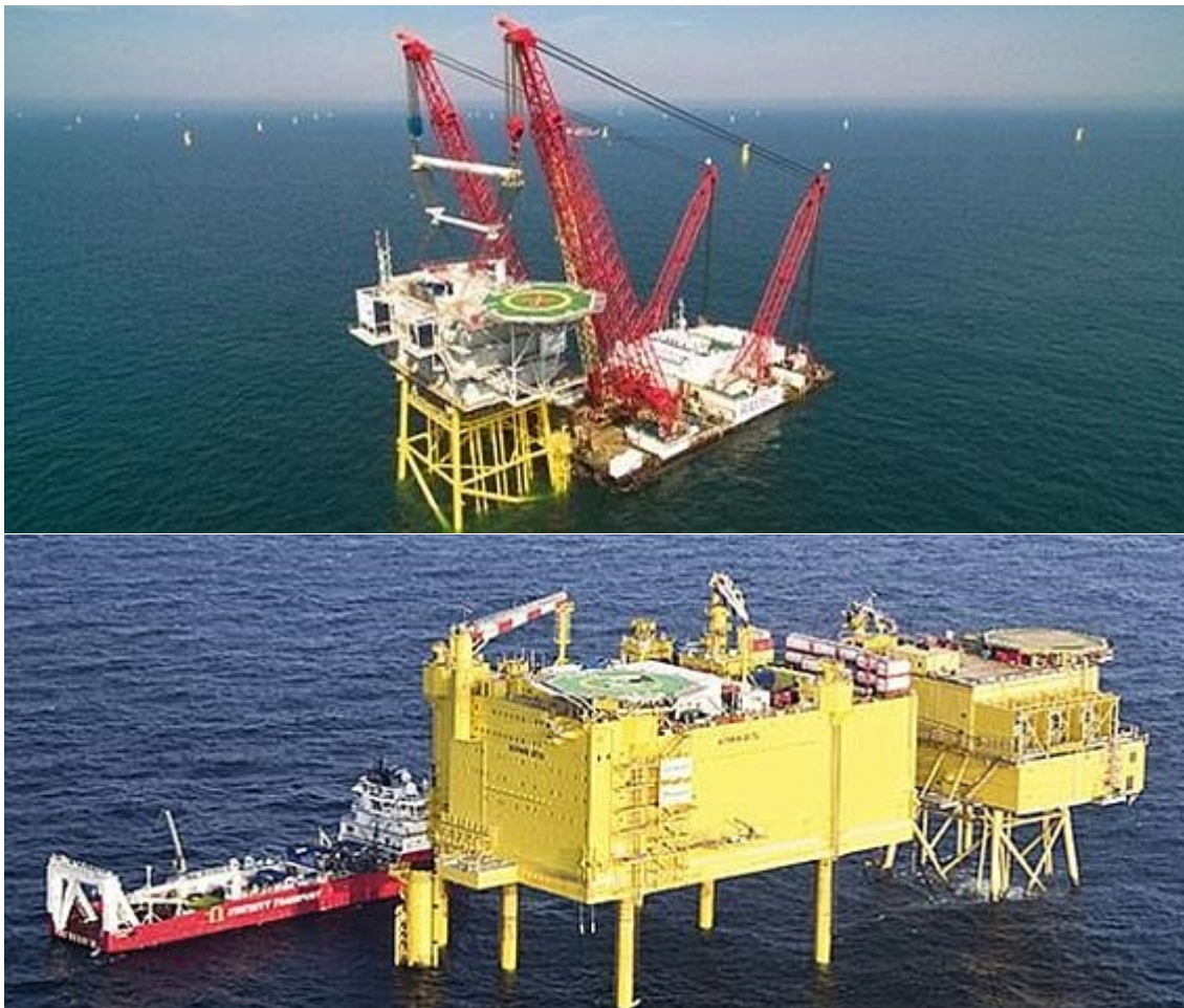
Figure 2-22: Offshore high voltage substations: (upper) 300MW HVAC platform installed at Gemini wind farm (Gemini, 2015), (lower) 800MW HVDC BorWin beta platform of TenneT TSO (Siemens, 2014)
