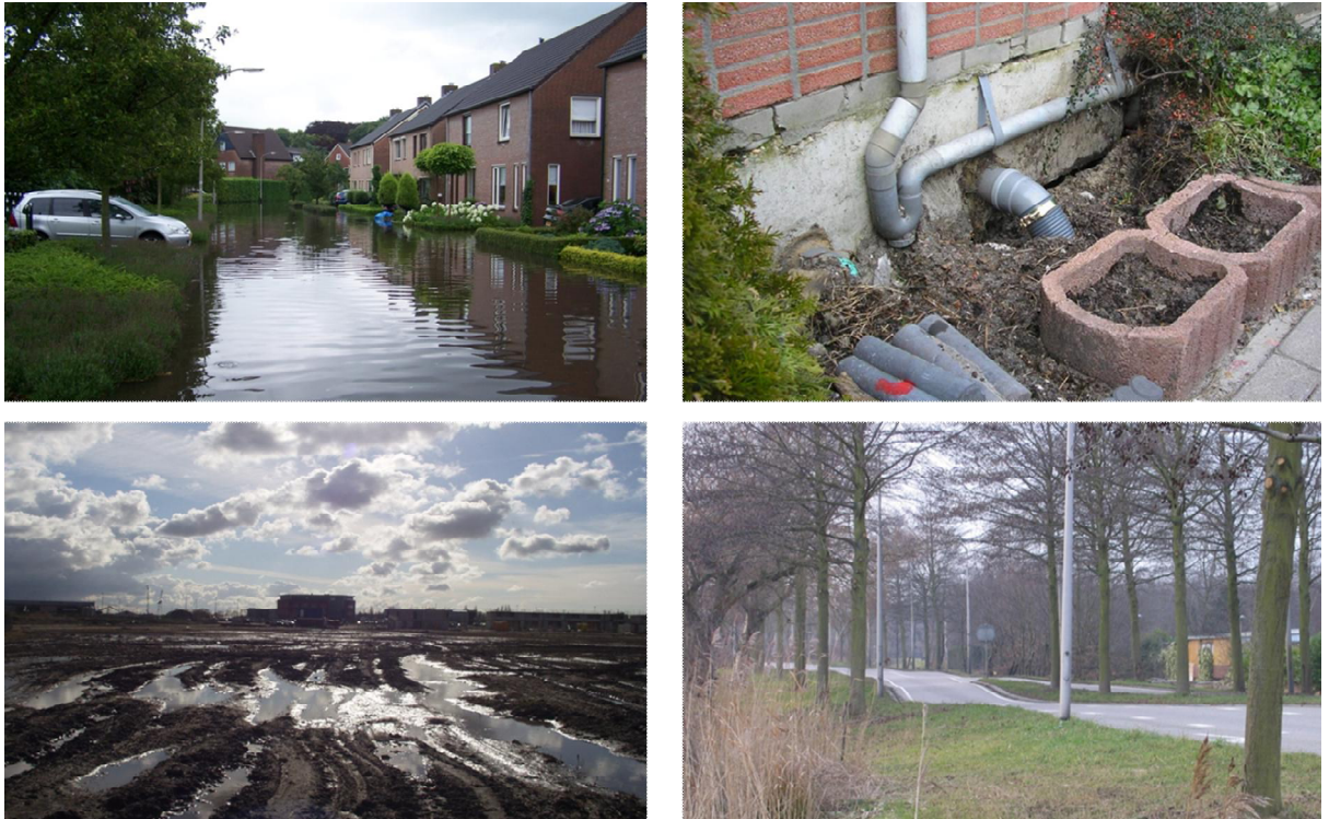
Figure 2.3 Some views of subsidence effects in soft soil regions in the Netherlands
