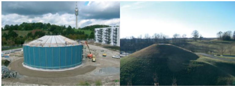
Figure 2: Large hot water storage combined with solar thermal district heating in Munich, Germany
