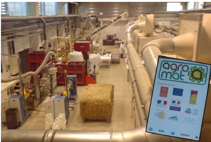
Figure 2: View of the Agromat demonstration building in Tarbes
