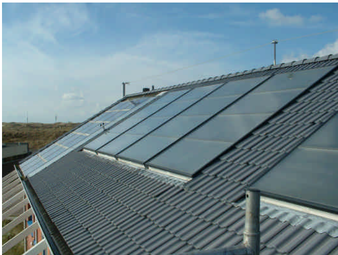
Solar thermal and PV panels on the ECN Research Dwelling roof
