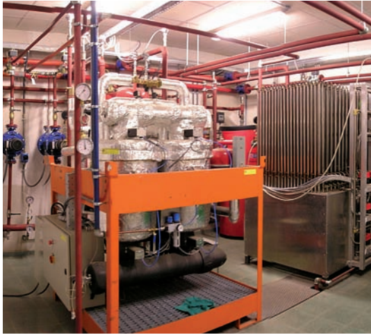
SOCOOL sorption cooling machine at Fiat-CRF.
