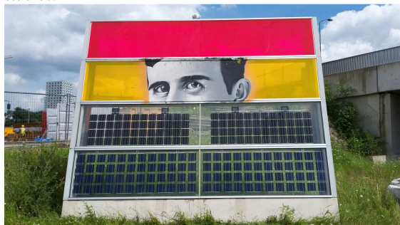
Figure 7: Depiction of the PVNB after the removal of the graffiti.
