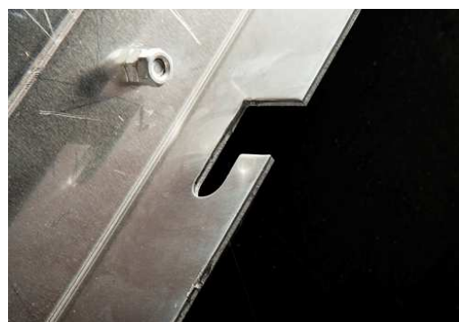
Figure 11: Rear side of the façade elements showing the Aluminum frame for mounting the modules to façades.
