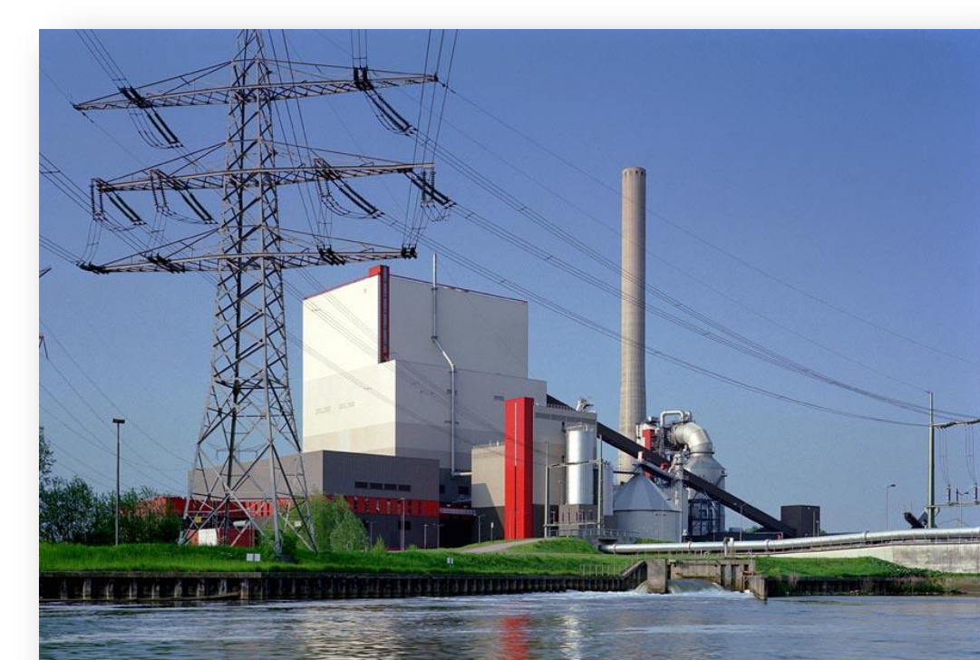
80 MW th CFB gasifier, Amercentrale 9 plant, Geertruidenberg, NL
