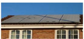
Figure 1: Residential PV system shaded by a lighting
