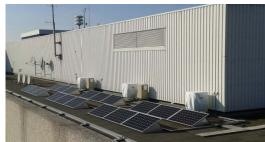
**Figure 3**: Impression of the field test. Every PV system consists of two successive rows of three solar panels. On the right side is the micro inverter system while in the middle is the reference string inverter system. On the far left is the power optimizer system. The measuring equipment and inverters are located in the cabinets behind the panels.
