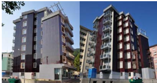
Figure 2: Palazzo Positivo after the retrofit. The whole façade is covered by BIPV (source: Frontini, SUPSI)
