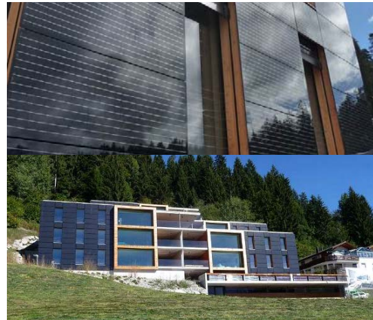
Figure 3: Casa Solara in Laax (Switzerland). The façade is clad with BIPV and wood (source: MGT)
