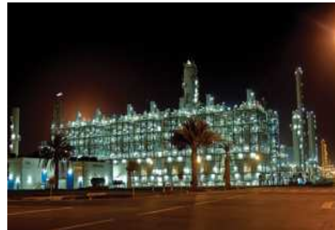
Recent startup of the largest ethane cracker - 1.5 mtpy ethylene, $1.3 bn (Source: Hydr. Proc. 2012).
