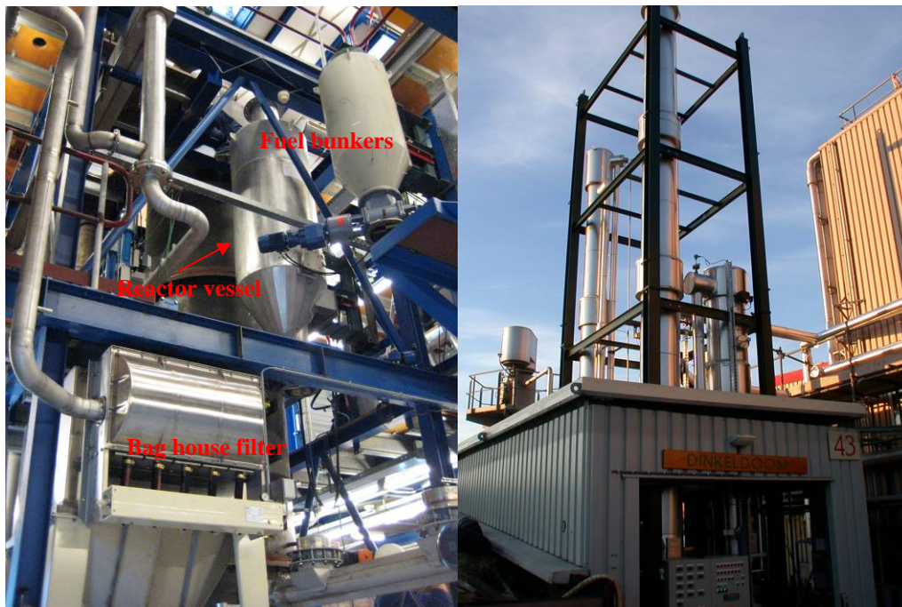
Figure 5. Photos of Pilot scale MILENA (left) and OLGA (right) installations
