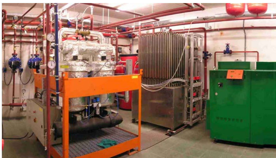
Figure 4: Picture of adsorption cooling prototype system integrated in the tri-generation system of the ECO-canteen of CRF (Italy)
