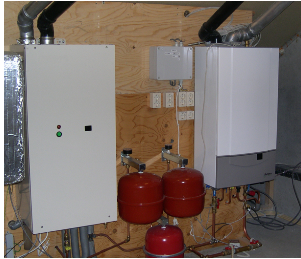
Figure 1: Heat pump prototype (with HE boiler on the right)
