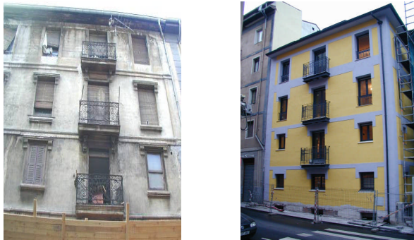
Spanish renovation project in Bilbao. Before and after renovation
