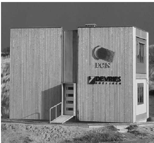
Figure 1: Above the four single-family dwellings and below the rotating test facility
