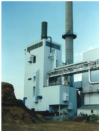
40 MW Burlington, USA
