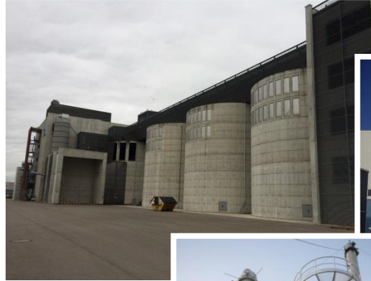
14 MW Senden, Germany
