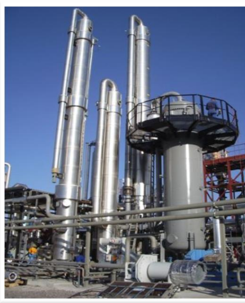
2 000 m 3 /h connected to updraft
