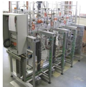
Further gas cleaning
