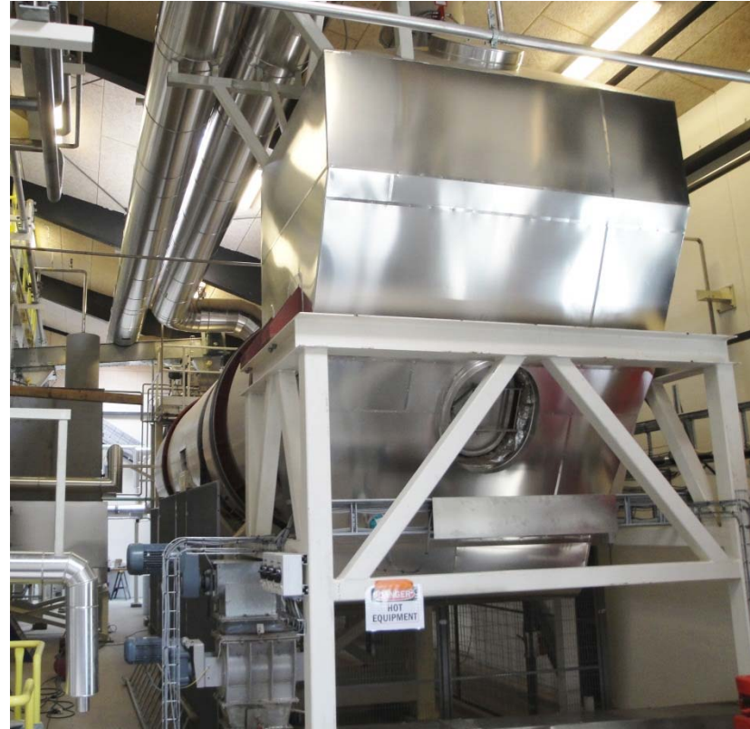
Viewed from Discharge End
