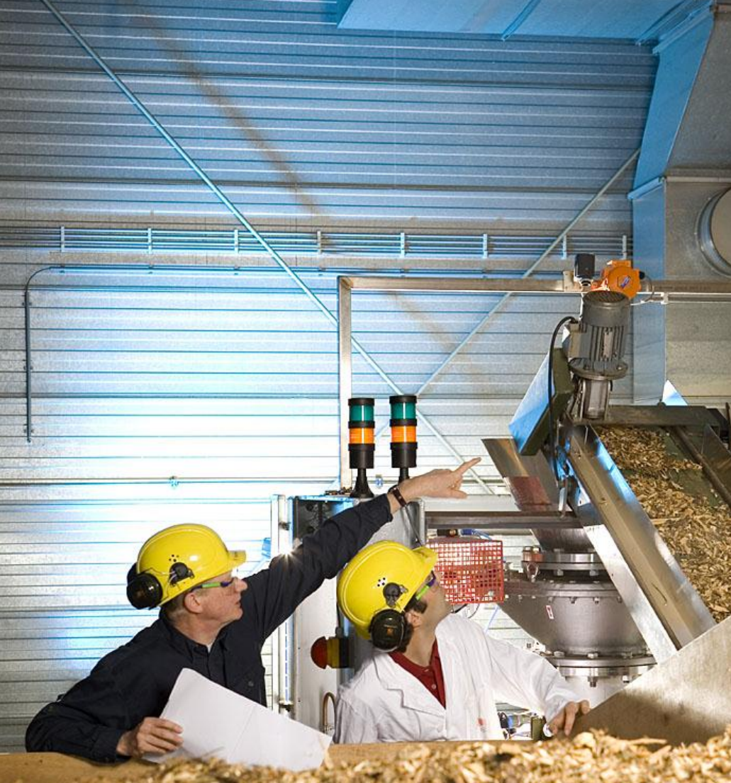
ECN 50 kg/h torrefaction pilot plant (Since February 2008)
