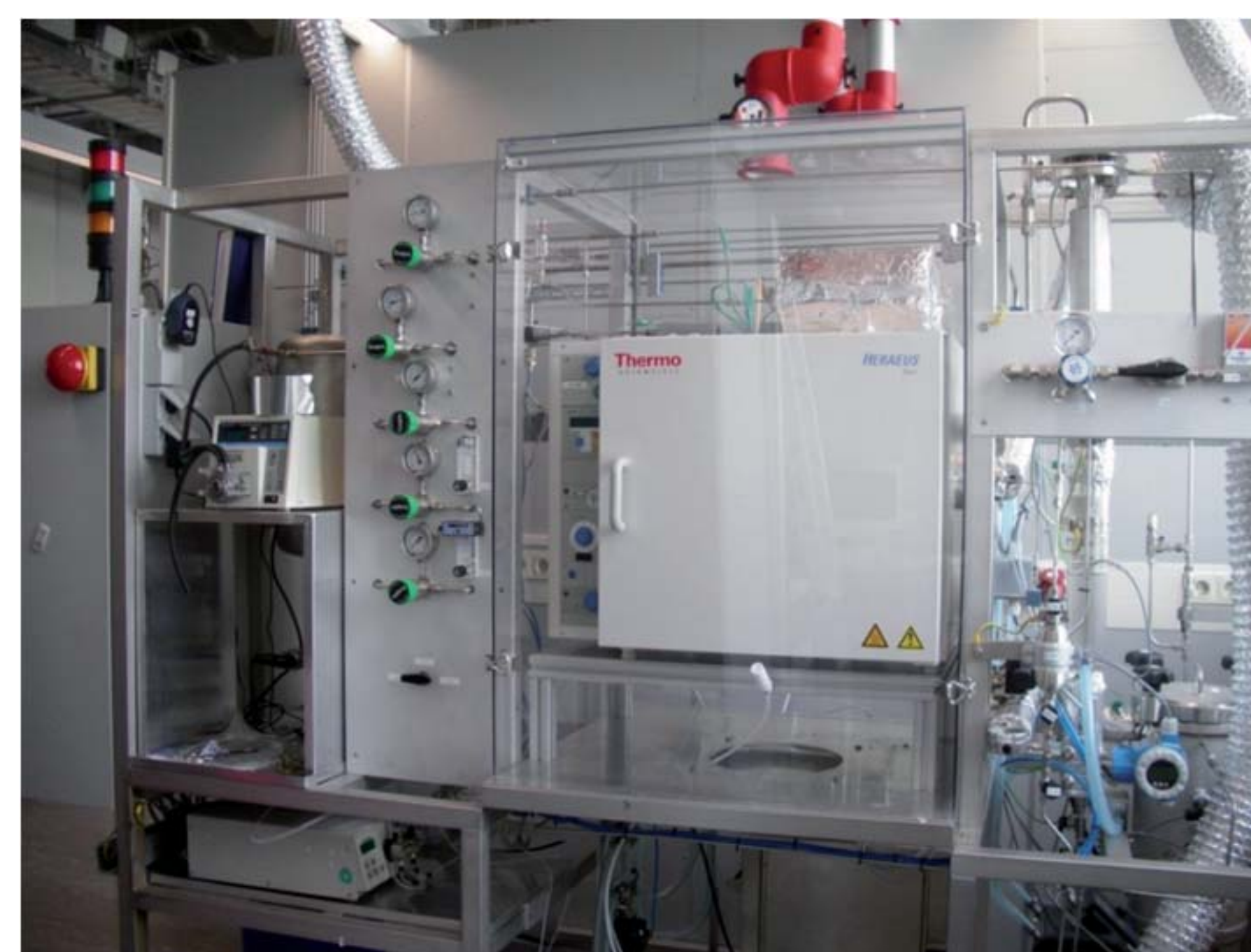
Figure 7: Taylor flow reactor installation build at ECN
