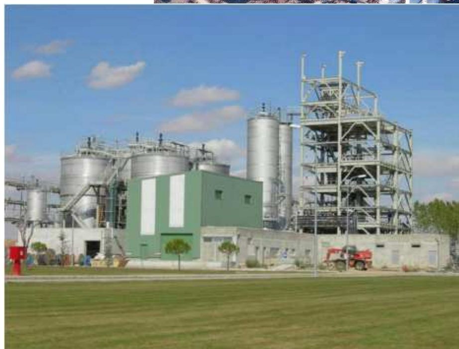
BCyL cellulose ethanol pilot plant AB, Salamanca, 5 Million L EtOH / year
