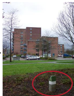
30 bar H 2 pipeline
