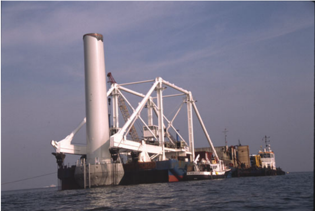
Figure 47. Special Installation barge for the gravity base support structure at Middelgrunden. When the barge is in place by Middelgrunden, several anchors are layed out, they are used to manouvre the barge so the turbine is in the right spot, it must be within 25 cm of the calculated position.
