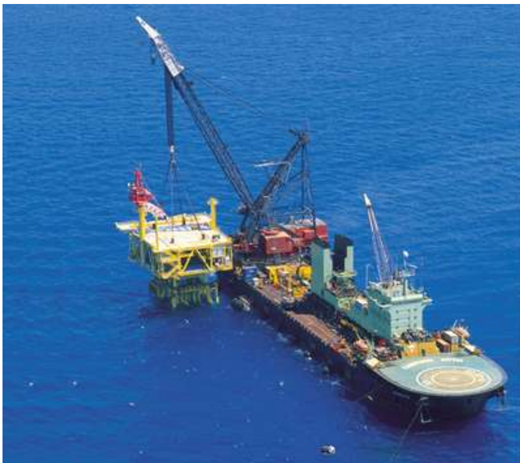
Figure 42. Typical Construction vessel.
