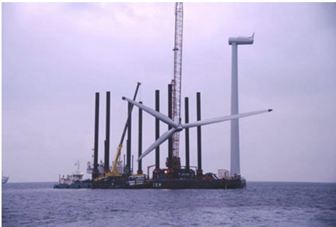
Figure 46. Installation of rotor at Middelgrunden wind farm. Wings and hub are raised horizontally until they can be tilted into vertical position. Then they are elevated to a height of 75 meters before they are mounted onto the nacelle. Source: Middelgrunden Internet site: http://www.middelgrunden.dk
