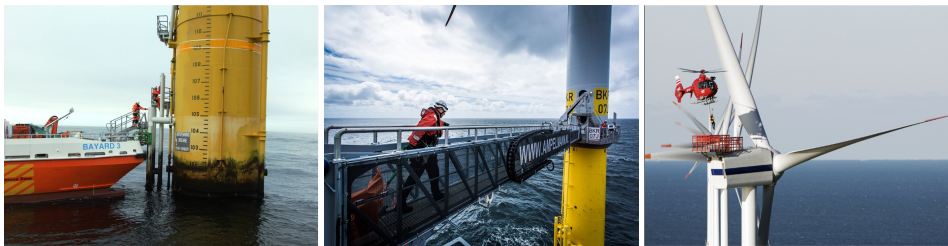
Figure 5: Access to the boat landing [4], platform [5] and helideck [6] (from left to right).
