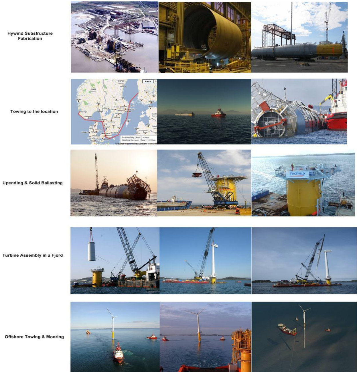
Figure 49: Planning steps followed during the installation of Hywind Floating offshore turbine [32]
