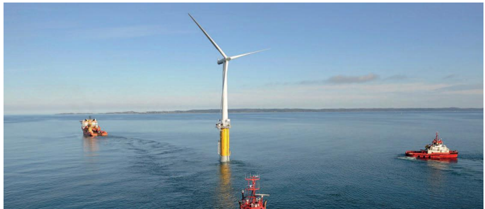
Figure 48: Statoil's successful Hywind floating offshore platform is towed into position. (courtesy Statoil)
