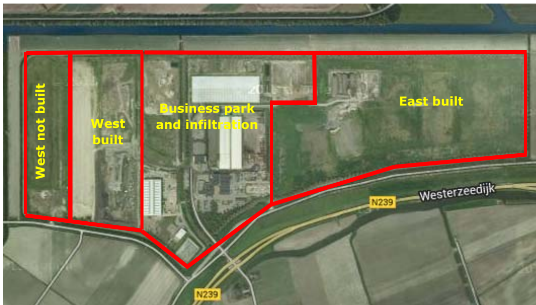
Figure 4.5: Aerial view of the Wieringermeer pilot landfill.
