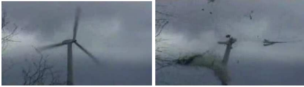
Figure 86 Snapshots of a movie of a wind turbine 'run-away'. As a result, the blades were torn away from the wind turbine.
