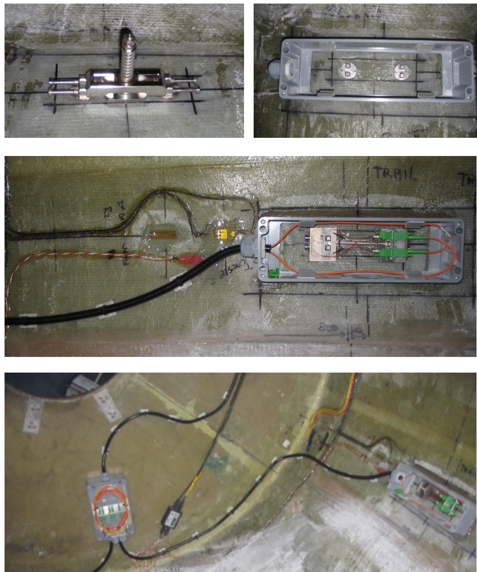
Figure 6.1: Instrumentation of the FOBM sensor assembly and the location of the electrical strain gauges
