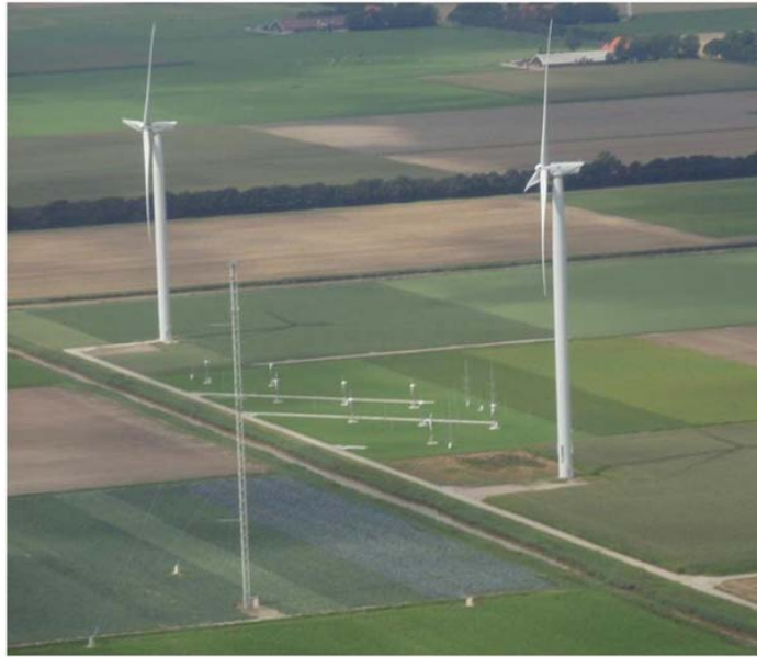
Figure 4 Scale wind farm on the EWTW, in between 2 prototype turbines and a tall measurement mast.
