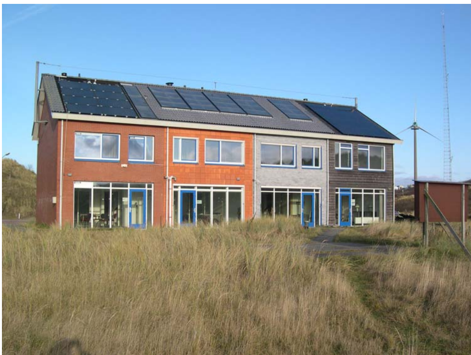
Figure 1.1 HV CIS modules on the roof of the most left Ecobuild house A, and a-Si modules on the roof of the most right Ecobuild house D [ECN]
