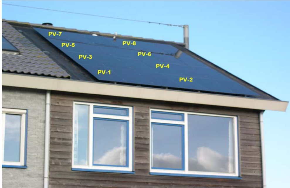
Figure 3.4 The a-Si modules on the roof of Ecobuild house D including references [ECN]
