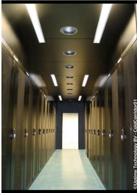
Figure 4.2 Situation where cold and hot air are kept separate. Photo: UpTime Technology
