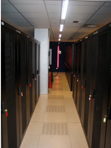
Figure 2.2 Computer equipment stacked in racks in large spaces where heated and cooled air can mix. Photos: ECN
