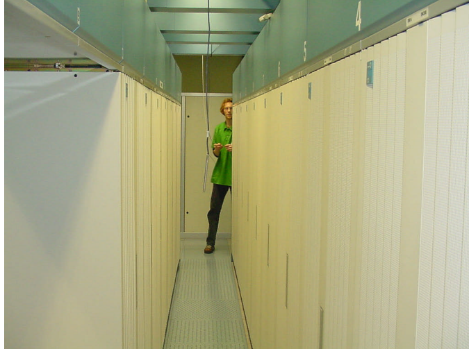
Figure 2.2 Computer equipment stacked in racks in large spaces where heated and cooled air can mix. Photos: ECN
