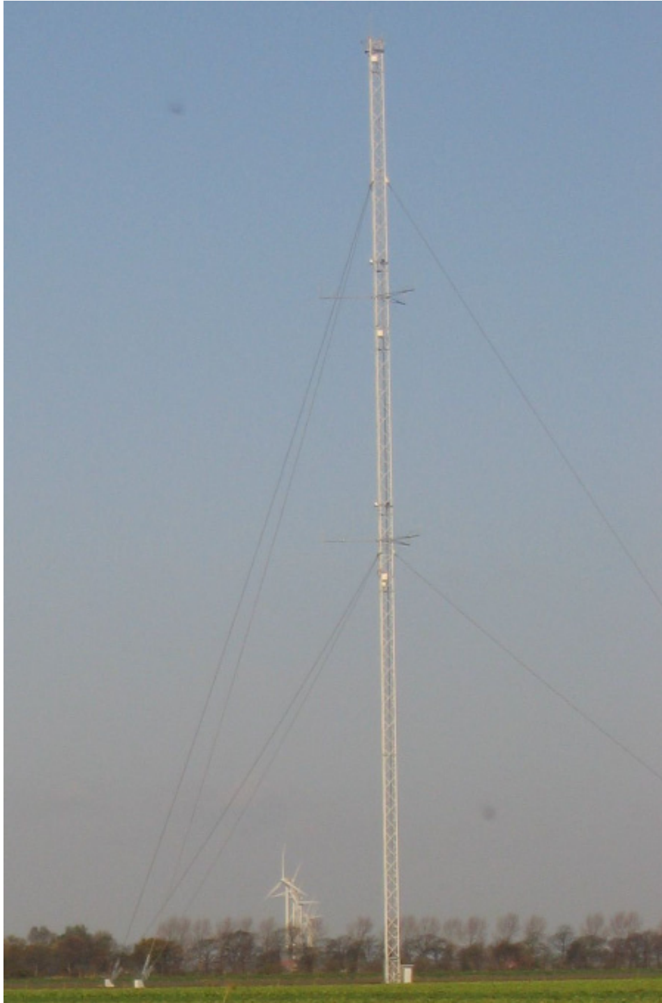
Figure 3.3 View of the meteorological mast 3 with attached booms at 50.4m and 78.4m heights and are directed to 0°, 120° and 240° with respect to North.
