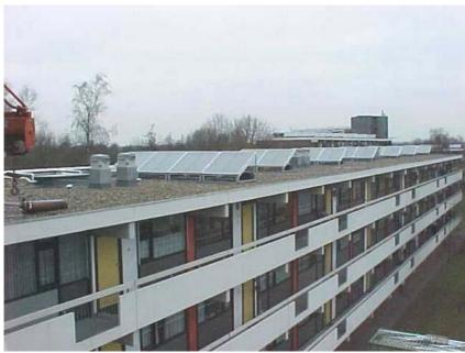
Figure A.1 Solar water heating system in apartment building in Veenendaal (NL)
