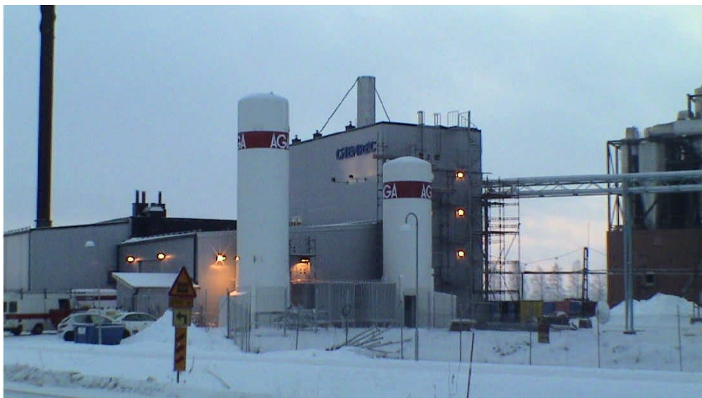
Figure 4.2. Chemrec black liquor gasification demonstration plant [40]
