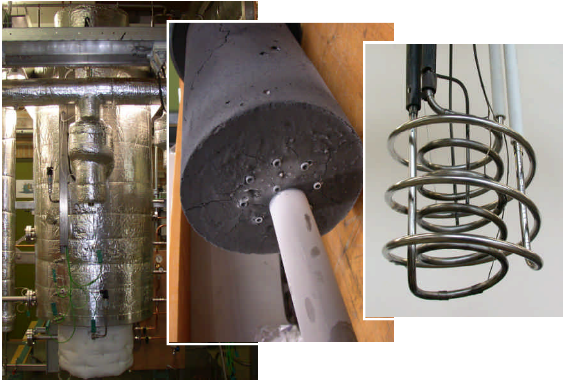
Figure 2.3. Picture of MILENA gasifier (left), upward view on refractory lined HELGA-reactor (centre), two cooling coils to be immersed in the HELGA fluidised bed (right)
