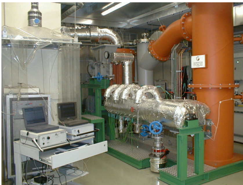
Figure B.3. The ECN pyromaat experimental facility
