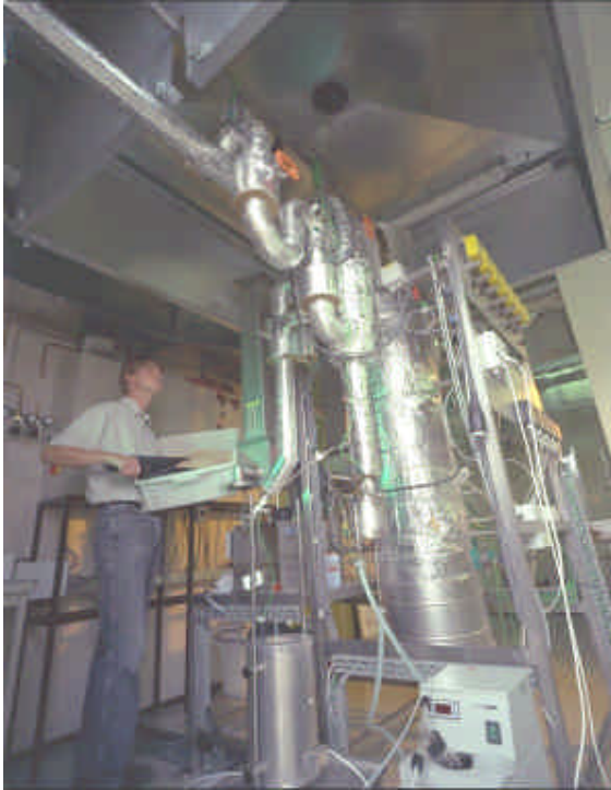
Figure 2.1 Photograph of the lab-scale fluidised-bed installation “WOB” at ECN
