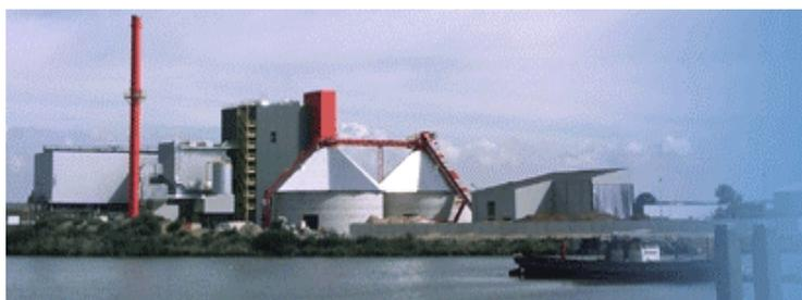
Figure 1.2 *80 MW<sub>th</sub> wood-fired BFB boiler in Cuijk, NL.*
