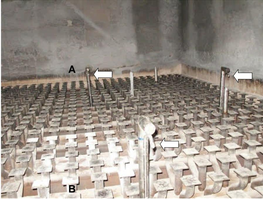
Figure 3.3 Photo showing three out of six pressure fluctuation measurement probes (section A-B from Figure 3.2).
