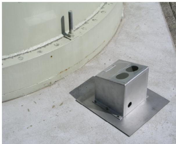
Figure 6.5: *Camera housing without mirror*
