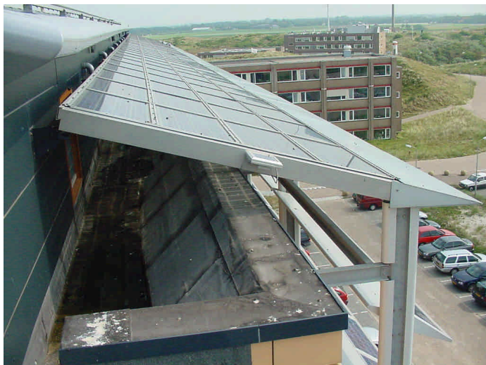
Figure 18 Photo of the support structure of the awning modules
