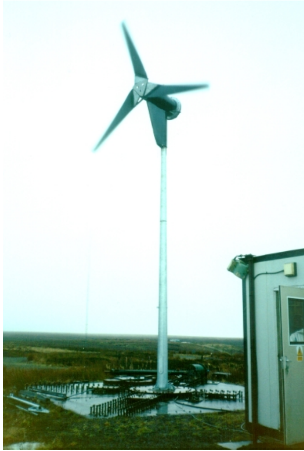
Figure 4: Proven turbine installed at NEL test site
