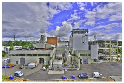
**Figure 8.8** The bioliq<sup>®</sup> plant at KIT: In a multistage process, high-quality synthetic fuels are produced from straw and other biogenous residues. (*Photograph: KIT/Tom Zevaco.*)
