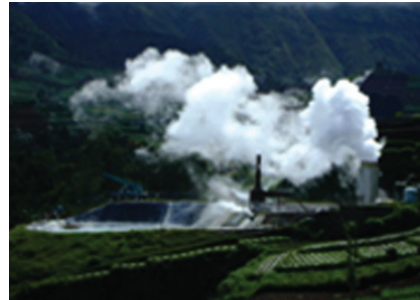
Figure 3.15 Geothermal Energy in Dieng, Wonosobo Regency, Central Java
