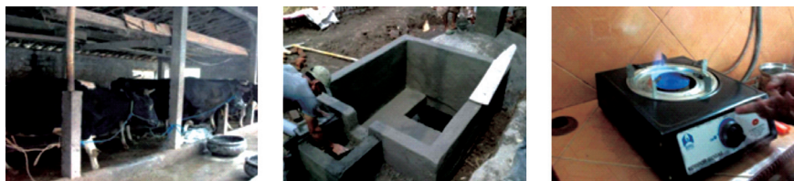
Figure 3.25 Biogas digester installed in Sruni village, Central Java
