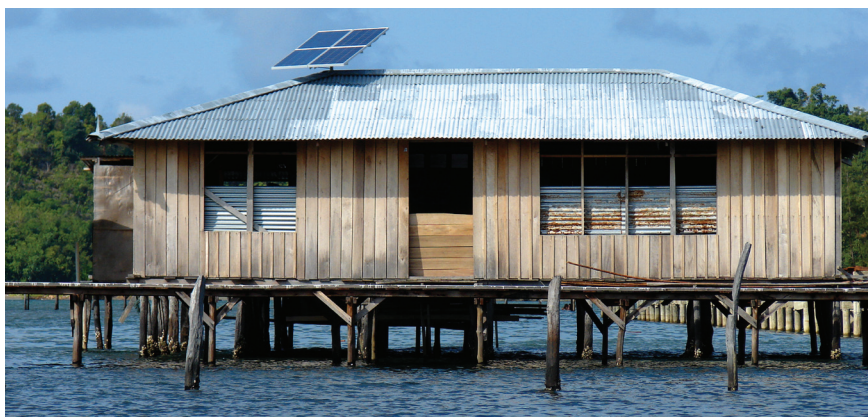
Figure 3.26 50 Wp Solar home system installed at home in Engross village, Papua.
