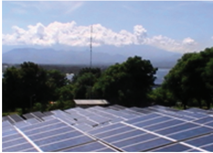
Figure 3.14 Centralized PV at Gili Terawangan, West Nusa Tenggara
