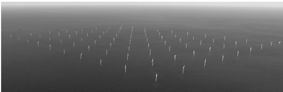
Fig. 17. 160 MW Horns Rev I offshore wind farm, consisting of 80 wind turbines of 2 MW each, near Esbjerg (Denmark). (Photo: Elsam, Vestas).
