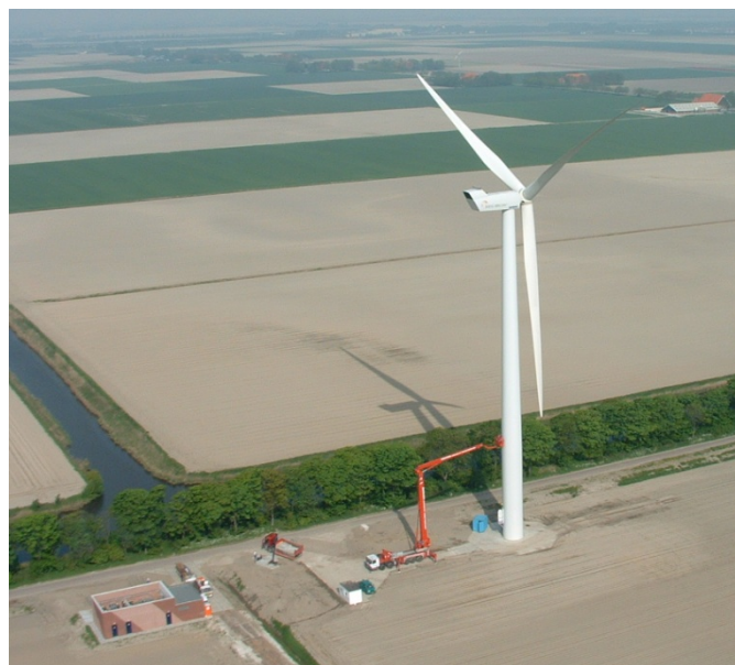
Figure 9-1: The NM90 2.75MW wind turbine (also known as DOWEC turbine) at the ECN test site in the Wieringermeer as seen from the measurement mast (109m) Source: [ECN, taken by R. Nijdam]
