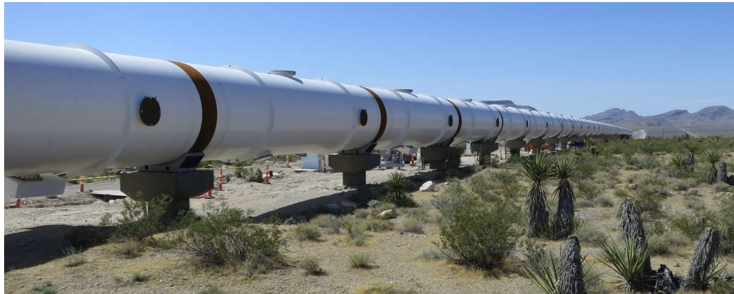
Figure 3. The 500 m long test tube of Hyperloop One in the Nevada dessert.
