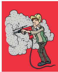
No protection measure Excess factor: 50 – 100 times
